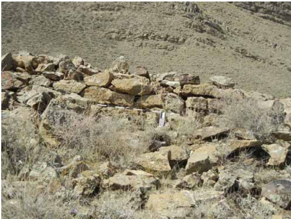
Figure 9: Photo of the 370-meter wall segment showing its internal face.
