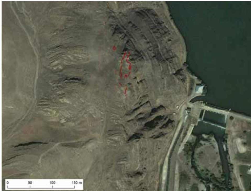
Figure 16: Plan of Qızqala 1 (ca. 0.6 hectare) for comparison to other mapped fortresses. Base imagery from Google Earth.
